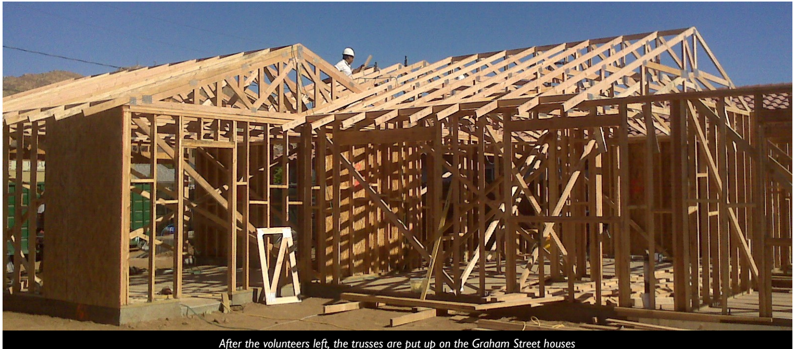
After the volunteers left, the trusses are put up on the Graham Street houses
